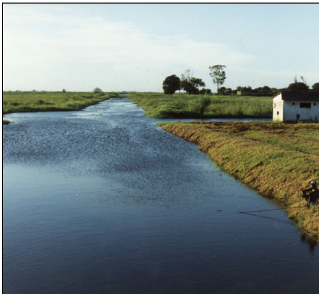
The Beira water supply intake and treatment plant are located 75 km upstream the river mouth
