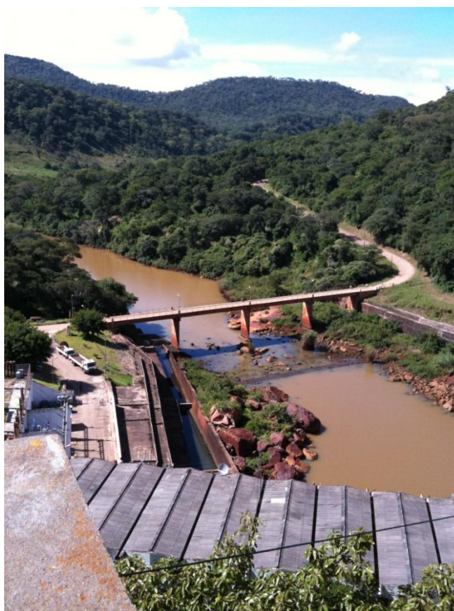
Figure 2-15 : View from Chicamba dam.
