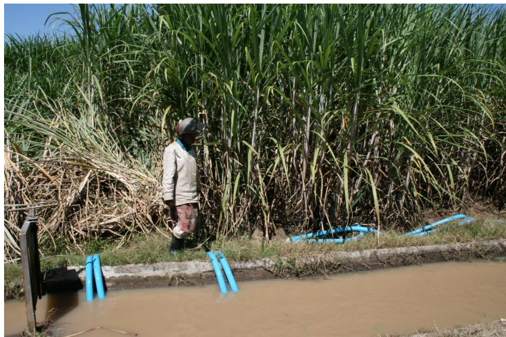
Figure 42 Irrigation in Triangle. The plots are supplied by siphons from concrete canals.
